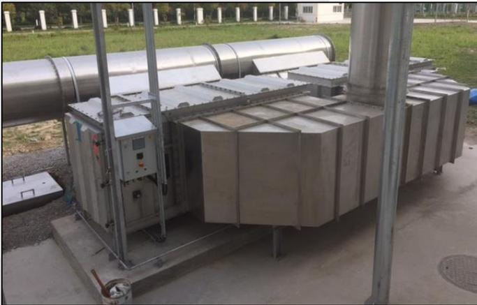
2V2-JHF-Belt Filters (twin set up) treating 55.000 m<sup>3</sup>/hr. vapor exhaust streams from an engineered plastic compounding facility.
