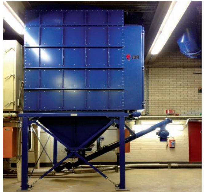
Depending on local legislation and plant conditions, alternatively mechanical filters (JOA-MII series) may be considered, due to the low dust loaded exhaust air from the MAX extraction.
