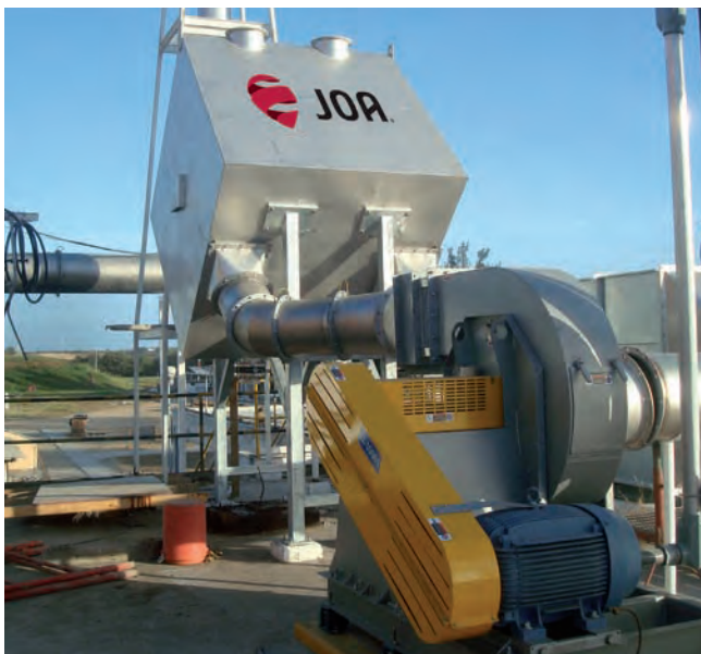
Low \Delta P -HEAF and Coalescer units combined with modular carbon bed odor abatement.
