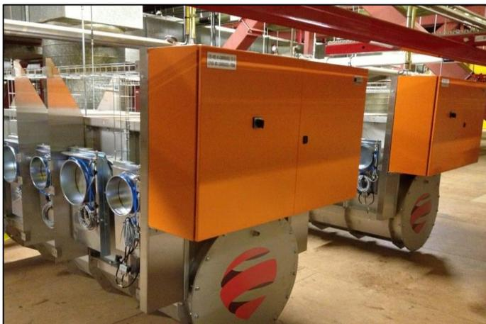
The JDF Dust Filter integrated with JOA Carrouseles for system balancing and full system flexibility for energy reduction purposes.
